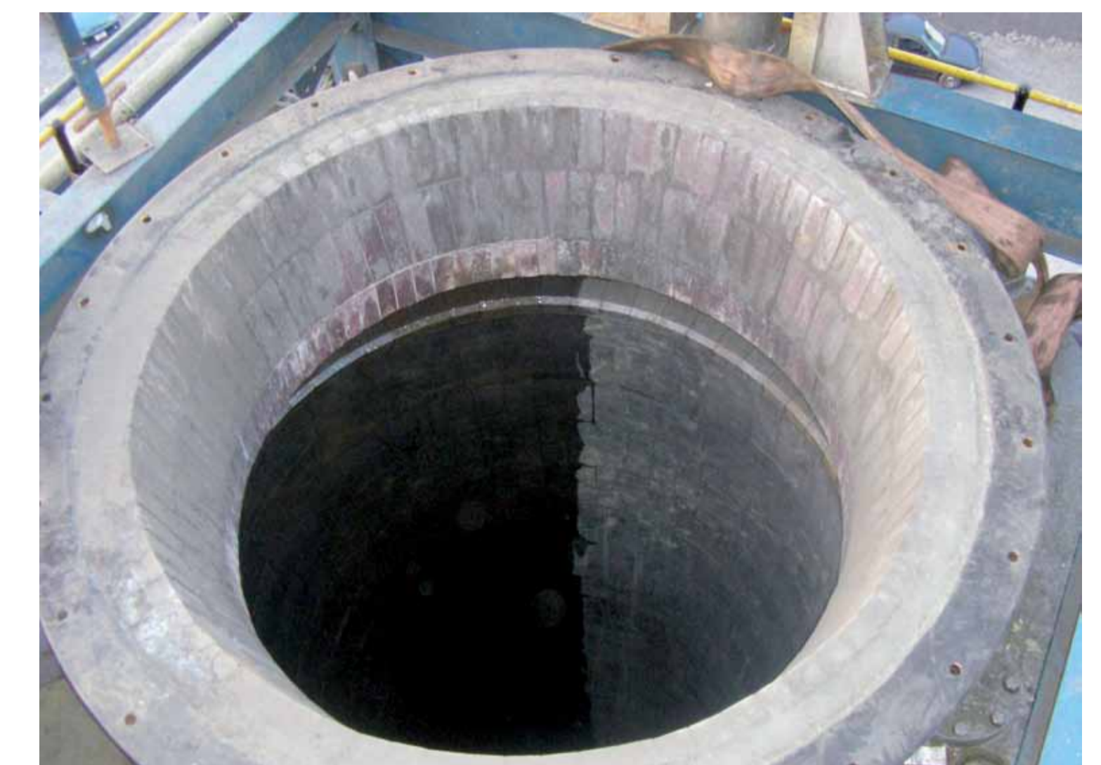
Transition piece: After installation and brick lining
